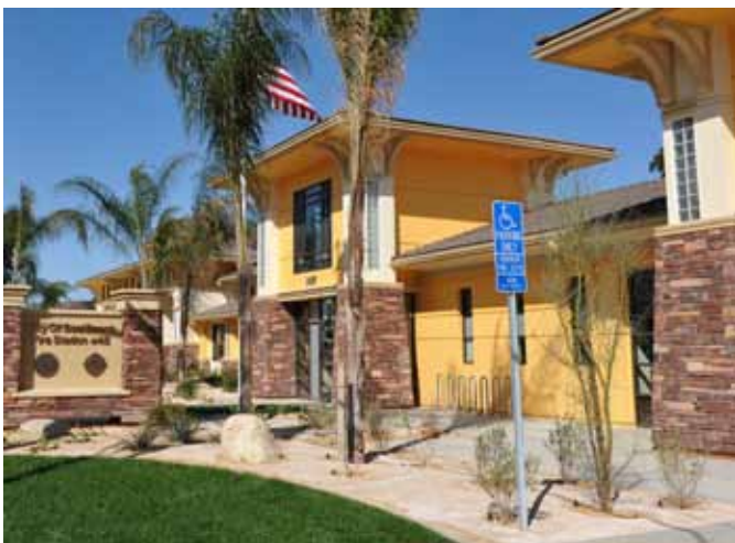
Fire Station 48 located in the City of Seal Beach
