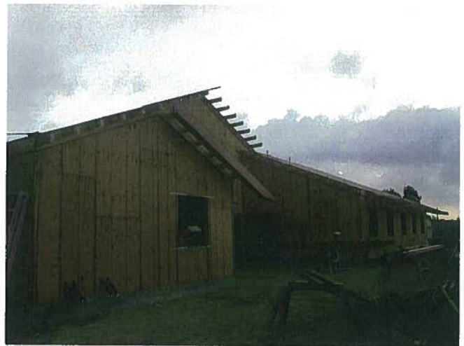
Construction of Fire Station 19 in Lake Forest
