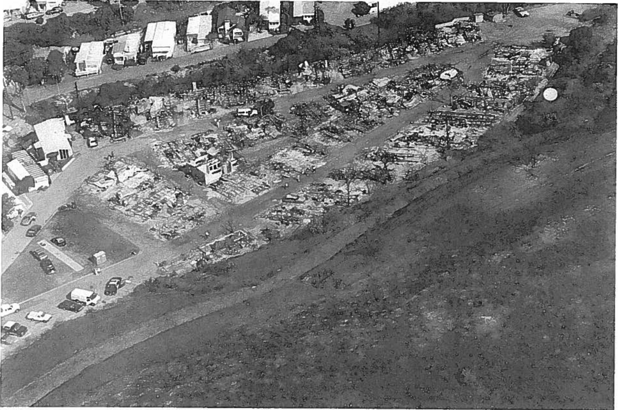
Destruction at El Morro Mobile Home Park. Forty-four homes in the mobile home park burned. Poor access due to narrow streets, limited water, and exploding liquid propane tanks complicated firefighting efforts.
