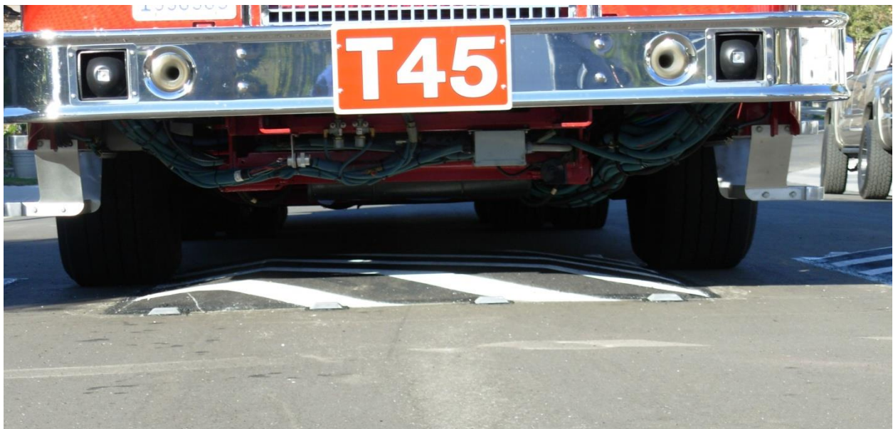
Figure 2: Fire truck straddling speed cushions. Locate the first speed cushion in the center of the street.
