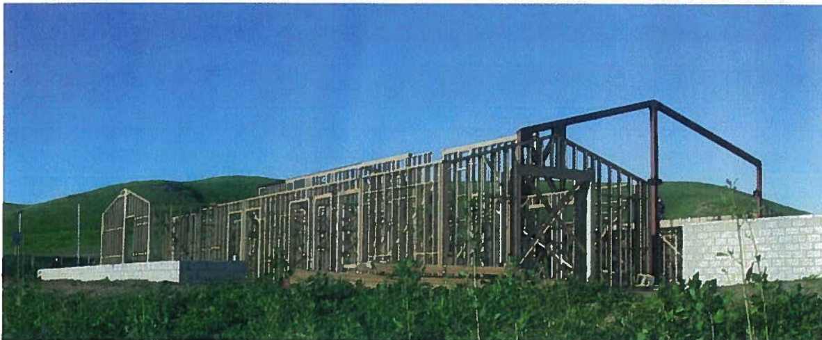
Fire Station 47 - Irvine
