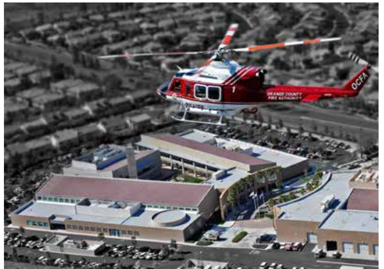
One of two Orange County Fire Authority Bell 412EP helicopters hovers above the OCFA Regional Fire Operations and Training Center.
